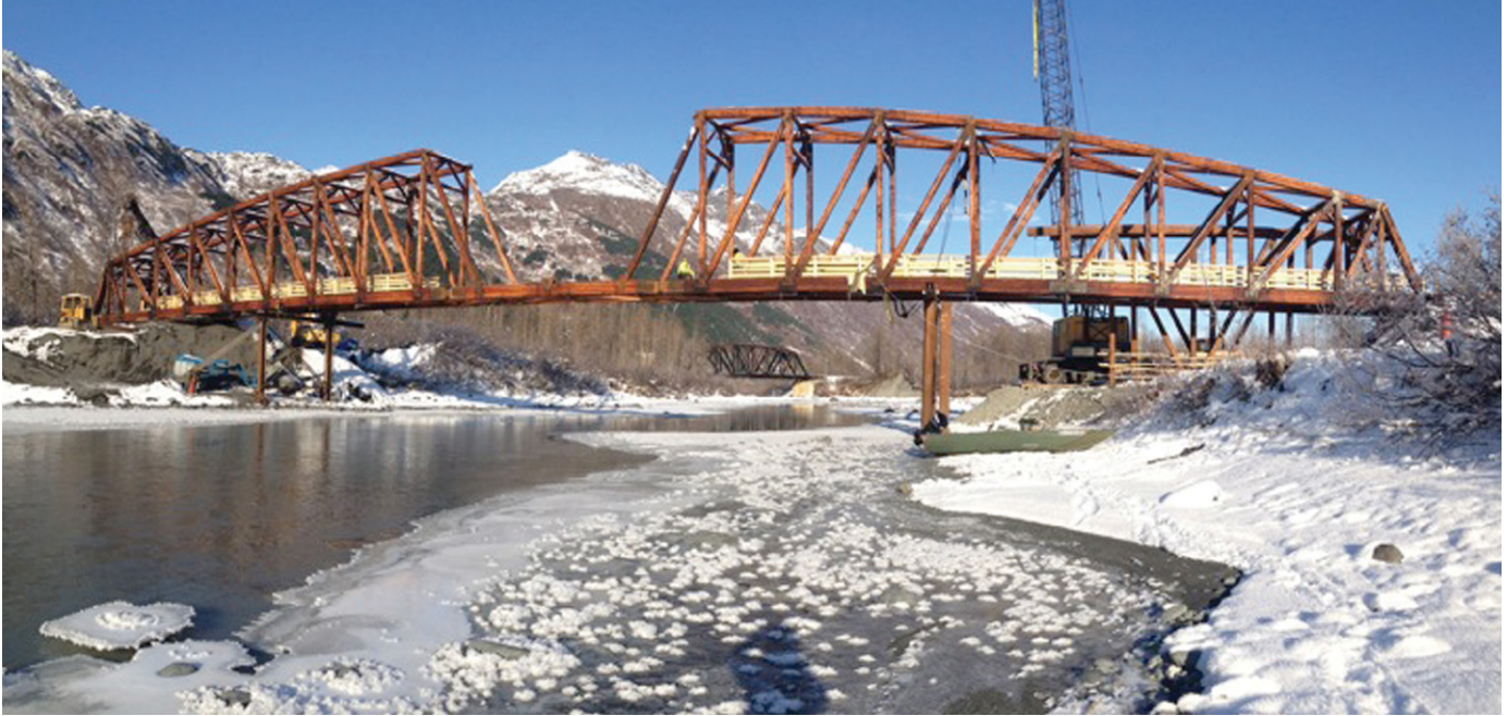
The bridge's 25-foot height eliminates the potential for collision with icebergs. Photo courtesy of USDA Forest Service.
