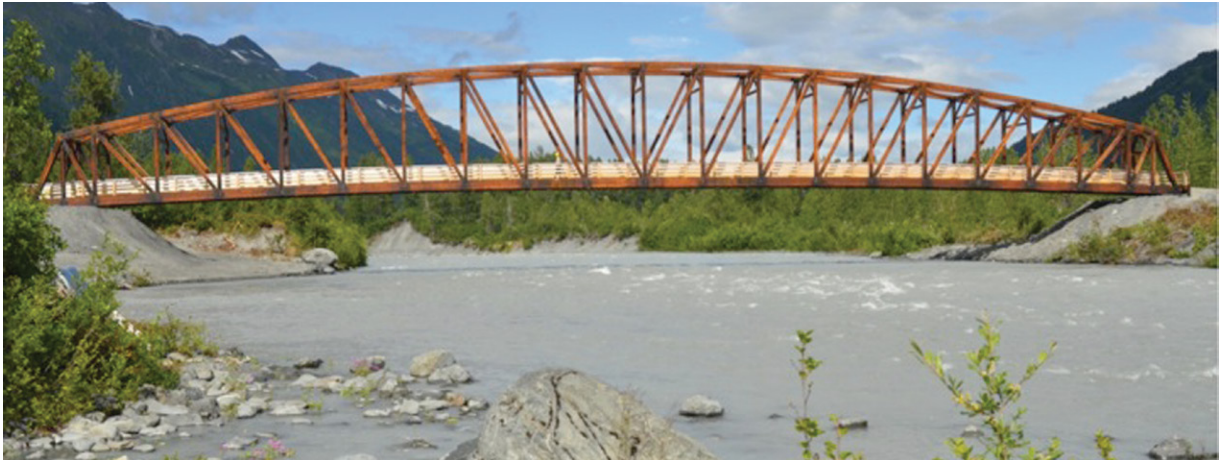
The 280-foot camelback truss bridge across the Placer River provides access to trails, camping, and scenery. Photo courtesy of Neil Hunt, Patrick Engineering.
