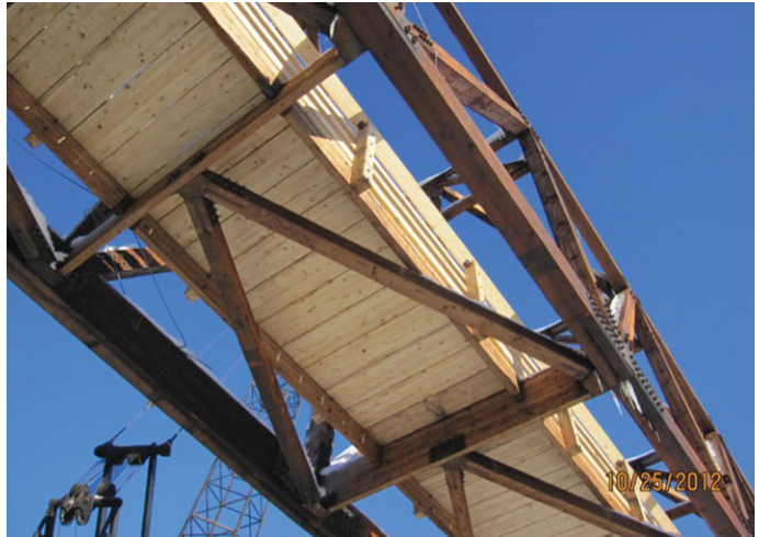
The deck and railing were made with Alaskan Yellow Cedar. Photo courtesy of USDA Forest Service.
