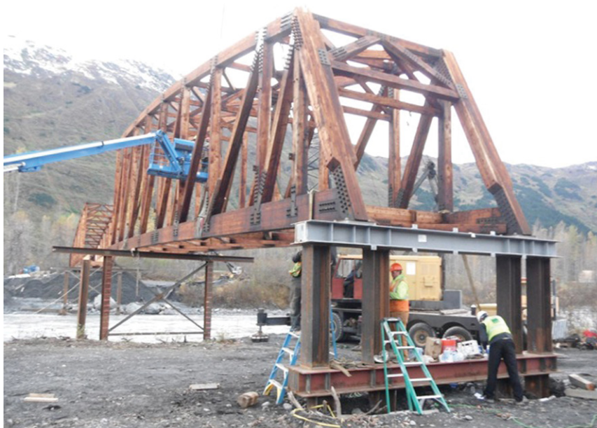
The bridge was constructed from both sides of the river. Photo courtesy of USDA Forest Service.
