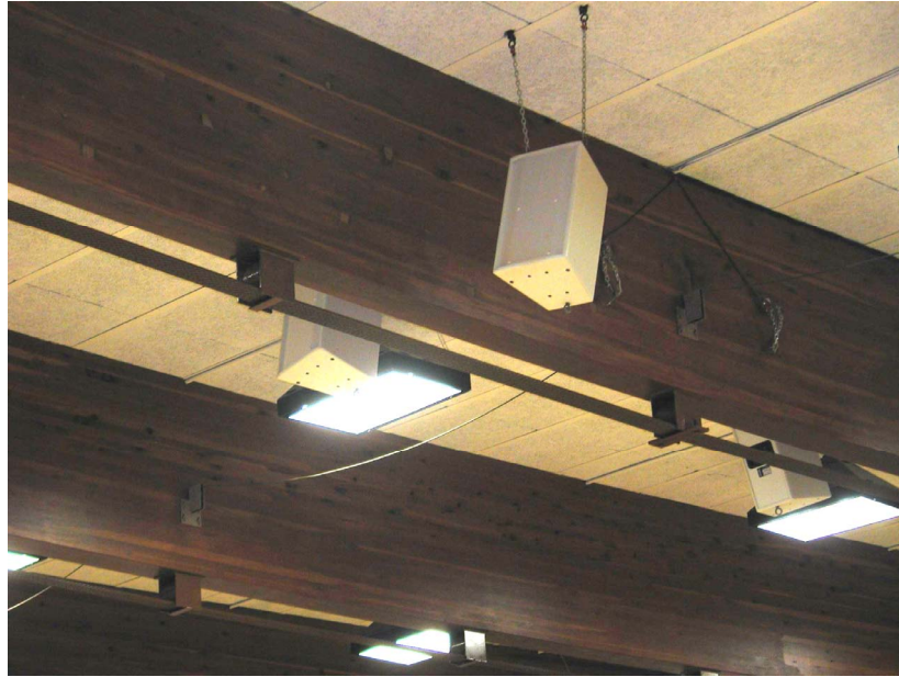
Figure 9. Completed repair/reinforcement of glulam girder beams.
