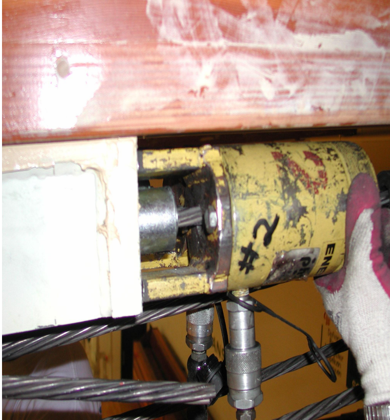
Figure 8. Head of hydraulic jack pulling on cable.
