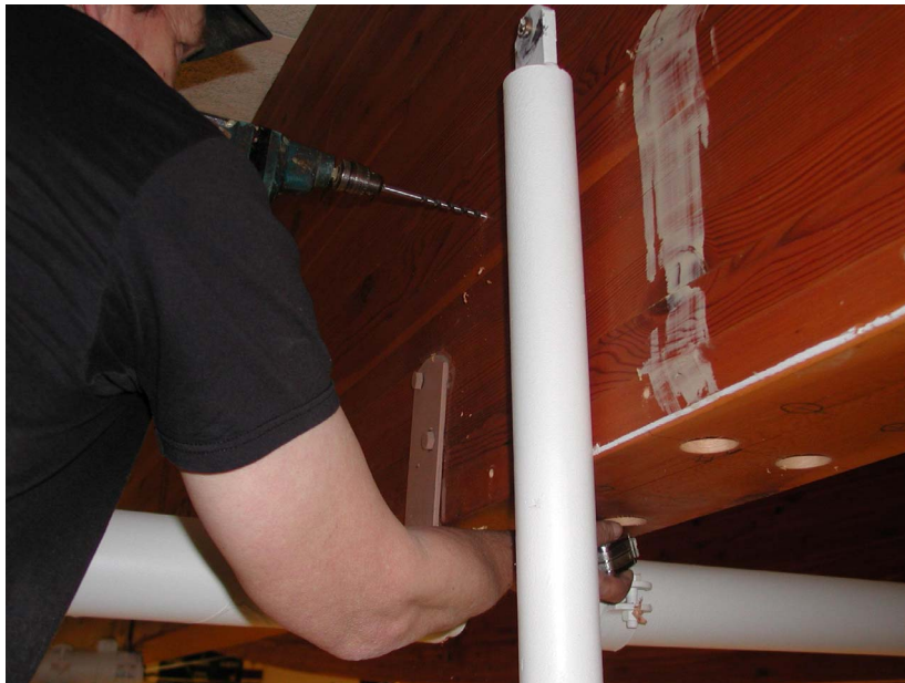
Figure 6. Drilling the injection and exhaust ports.
