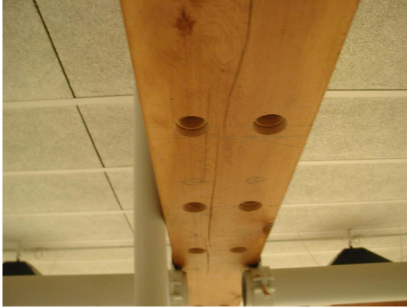
Figure 5. Holes drilled to receive Post-Tensioning Anchor Brackets.
