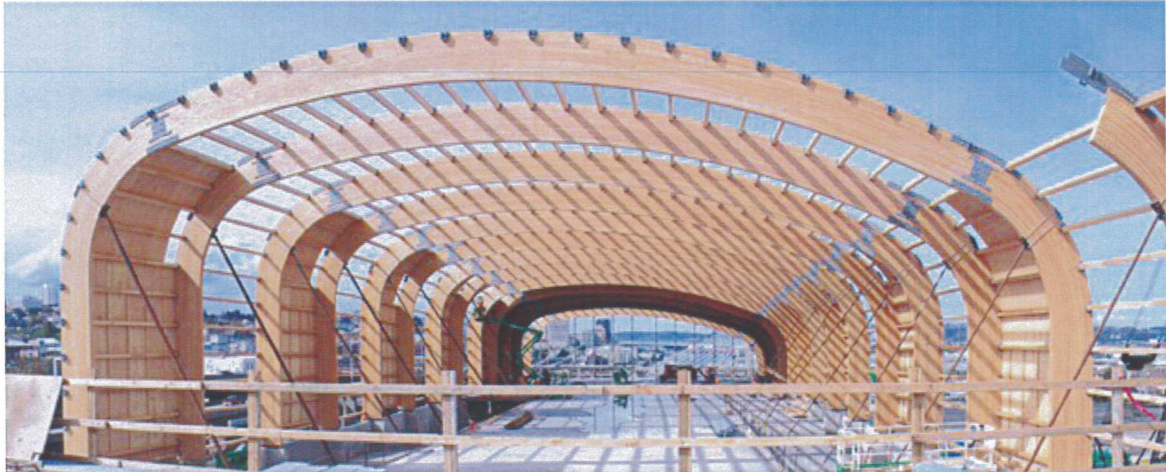
Glulam beams are erected to create the arched curve profile of the LeMay Museum roof, shown during construction in Spring 2011.
