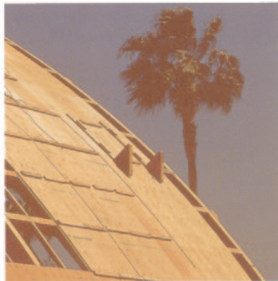
Bending the plywood by hand over the curved glulam presented a challenge.
