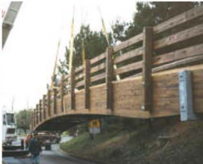
GREENWAY PEDESTRIAN BRIDGE BEAVERTON, OREGON
