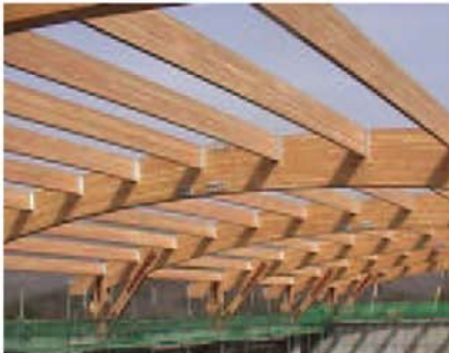
GYMNASIUM ROOF SOUTH KOREA
