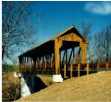
STONER CREEK BRIDGE PARIS, KENTUCKY
