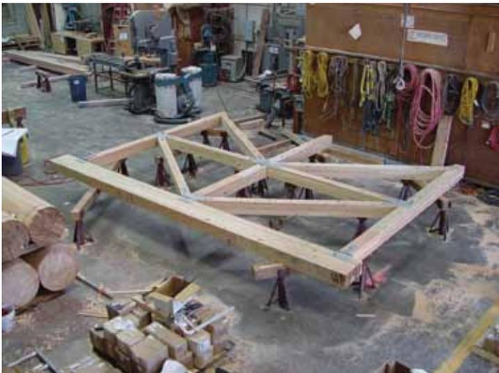
Figure 2: Pre-assembly of timber bents at fabrication.
