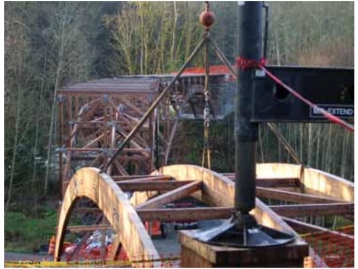
Figure 5: Bents on the center arch span are added and the northern arch span is set.
