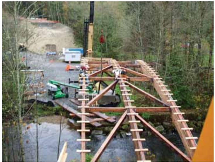
Figure 3: Installation of arch chevron bracing.
